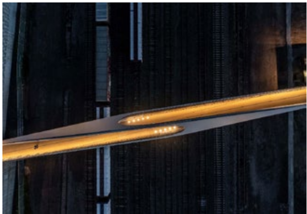
Jason O'Rear - Park Union Bridge 3rd Place in Architecture, Bridges
